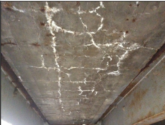
EFFLORESCENCE
